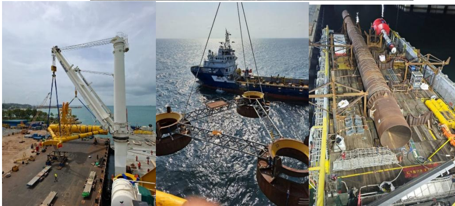
FLNG mooring job for Eni'S Congo LNG project; Source: GEOCEAN
