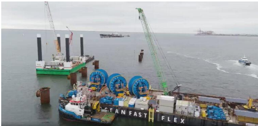
Installation of the PEM at Wilhelmshaven 2 LNG Terminal; Source: Geocean
