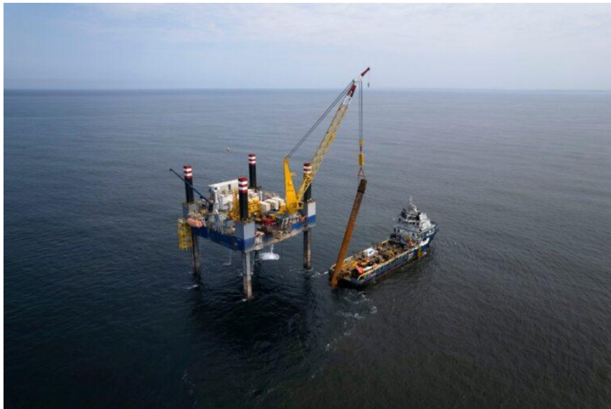
Casing installation; Source: GEOCEAN
